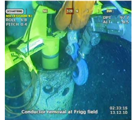
Connecting the crane hook to the stub
